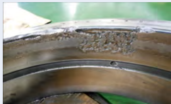
Fig. 6 Flaking damage on the outer-ring of a main shaft bearing
