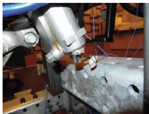
(f) An additional 3-axis accelerometer on the worm/wheel gear housing of steering column (No.9).
